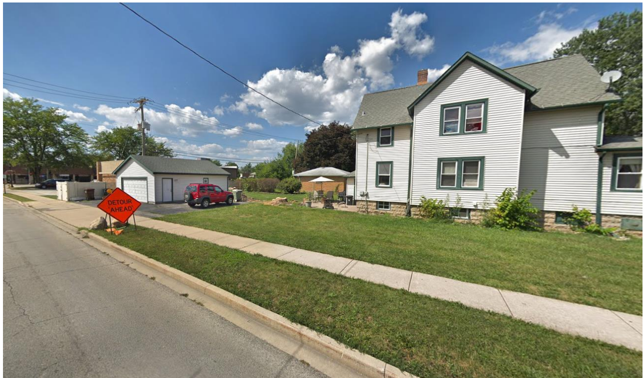
Above: Neighboring property to the north across 171st Street with a non-conforming accessory structure (garage).
