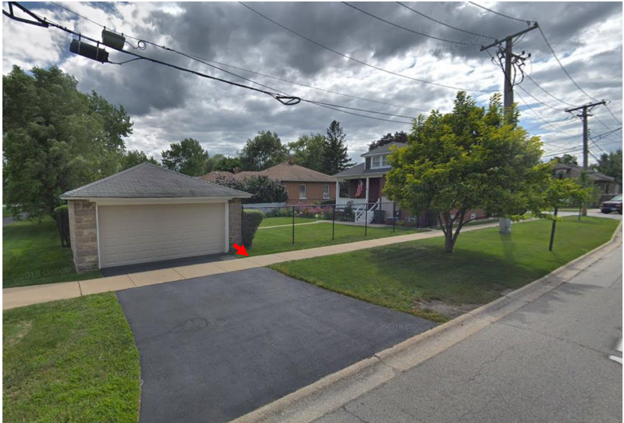
Above: Neighboring property to the east across 67 th Street with a non-conforming accessory structure (garage).
